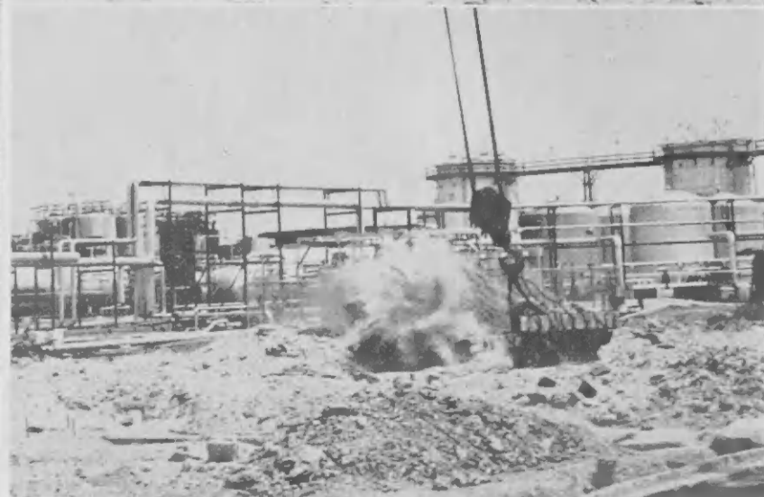
WITH A shove on the detonator, which sets up a high voltage current to a dynamite cap, top photo, M. Hazel explodes the charge. Off goes the dynamite, bottom photo, which destroys the concrete block.
